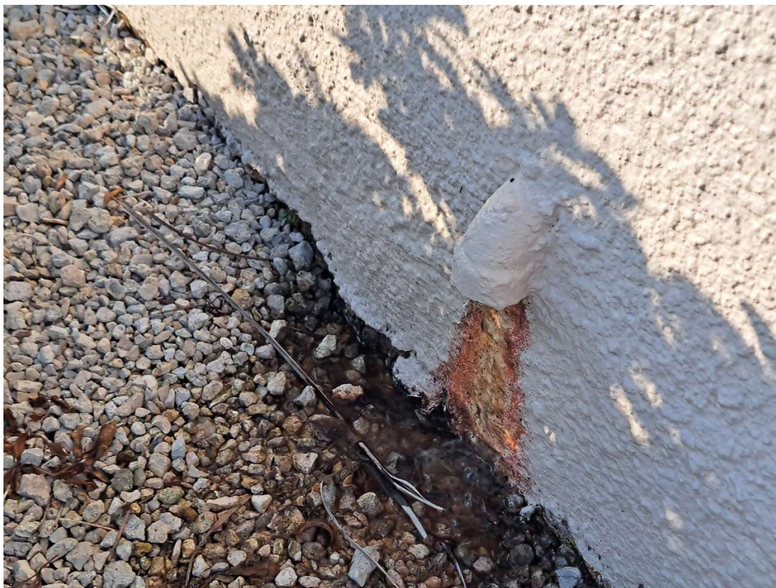
Photo 01 Ref: 2.1.1.1 – Downspouts Emptying Next to Foundations
