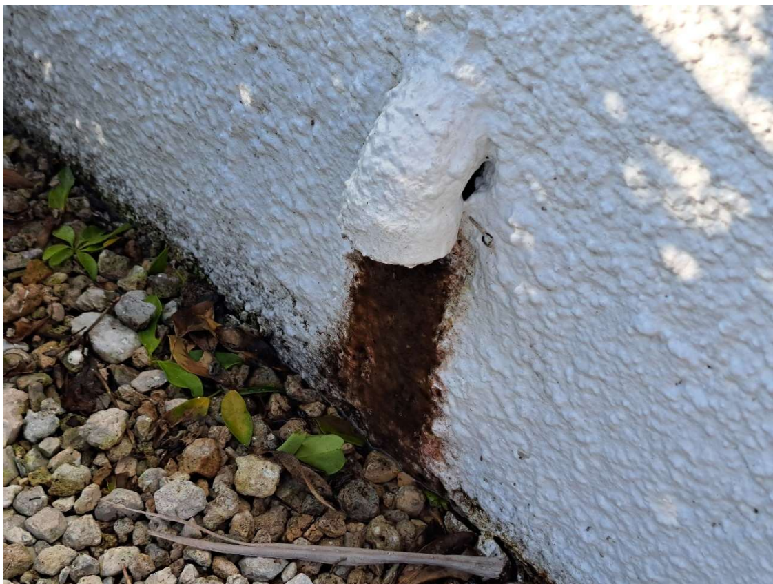
Photo 02 Ref: 2.1.1.1 – Downspouts Emptying Next to Foundations
