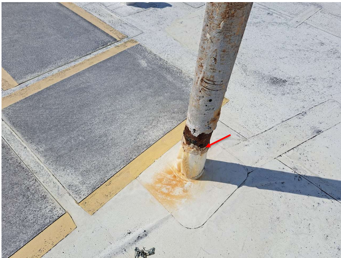
Photo 06 Ref: 2.1.3.1 – Damaged Upper Flashing of the Fire Hydrant Pipe on the Roof
